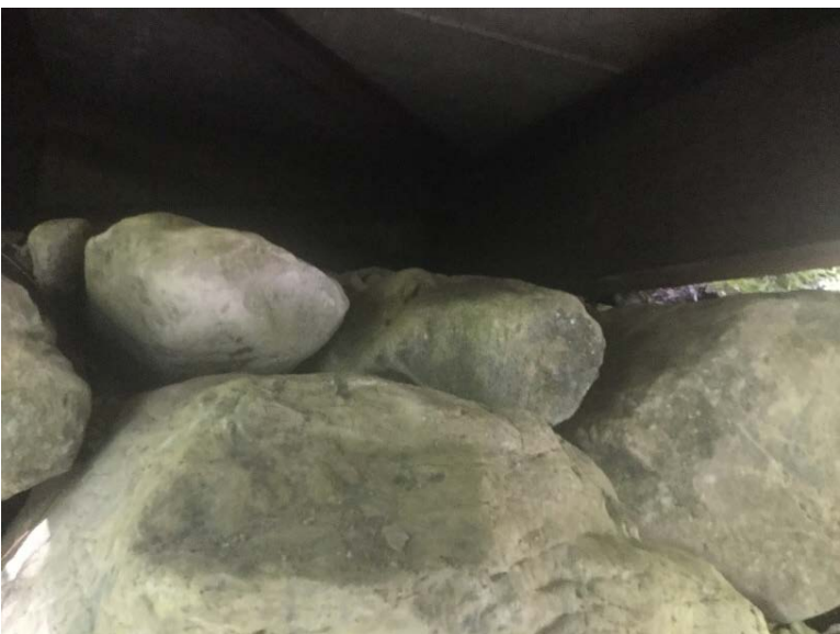
Right Bank Abutment when facing downstream
