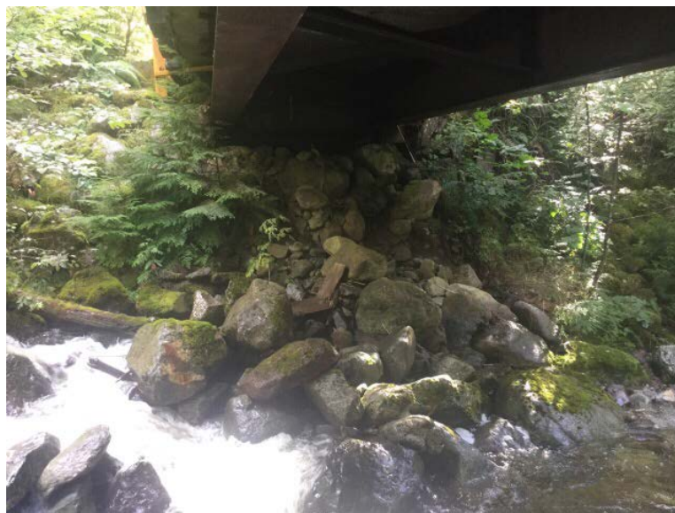
Left Bank Abutment when facing downstream
